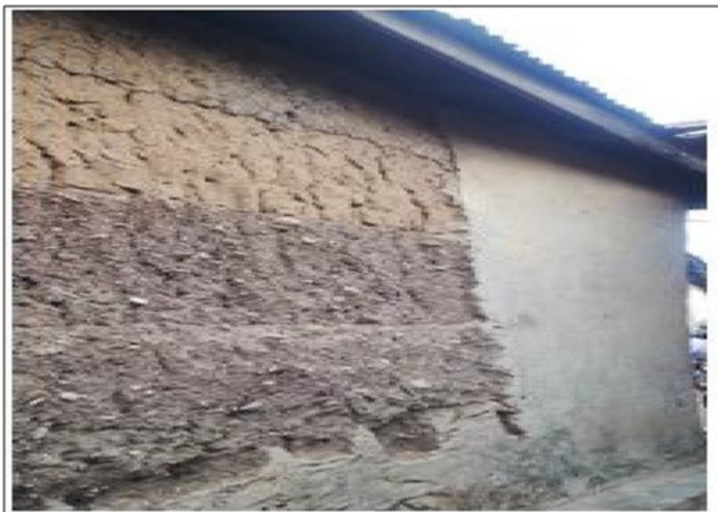
Plate 3: Cob wall/Direct layering wall construction partly rendered
