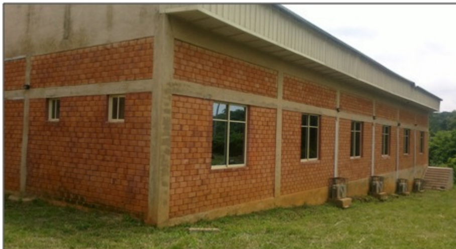
PLATE 6: A Building made of Compressed Interlocking Earth Blocks and Concrete Source: Taiwo and Adegboye, 2013
