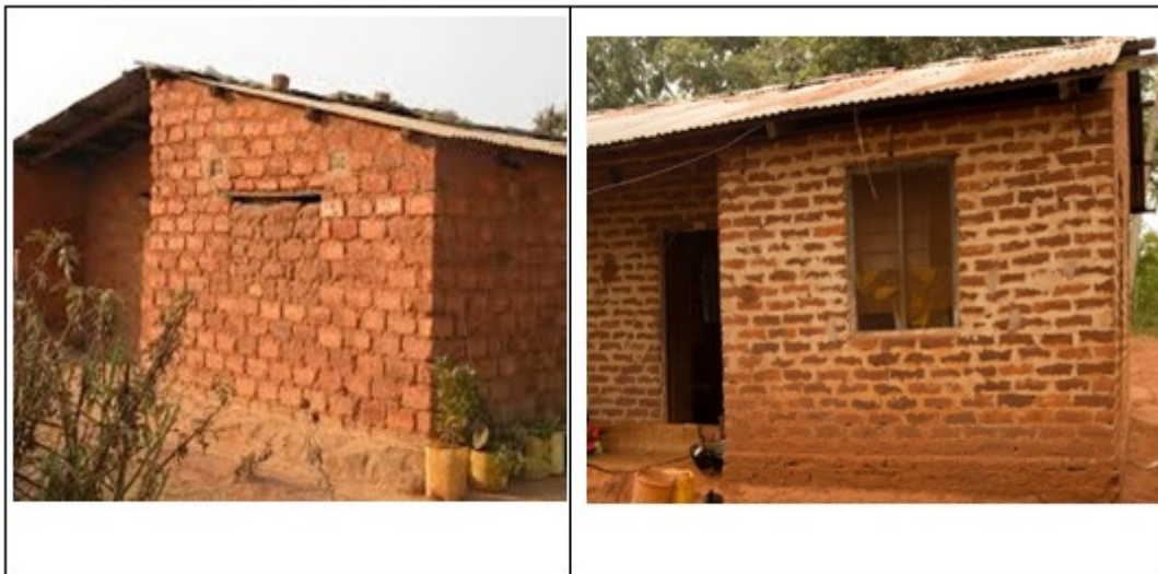
Plate 2: Adobe blocks coursed with soil and sand cement mortar joints.
