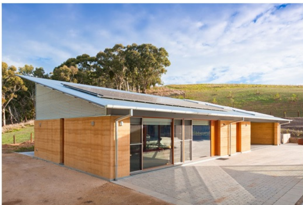
PLATE 9: Rammed Earth Residential Building Source: www.en.wikipedia.com
