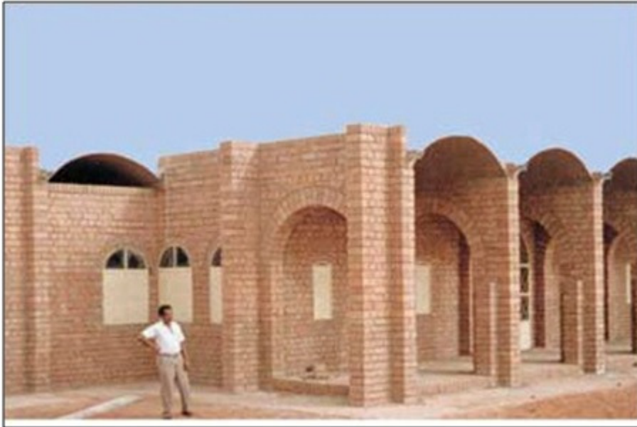
PLATE 7: A Building made of Compressed Stabilized Earth Blocks Source: Adam and Agib, 2001
