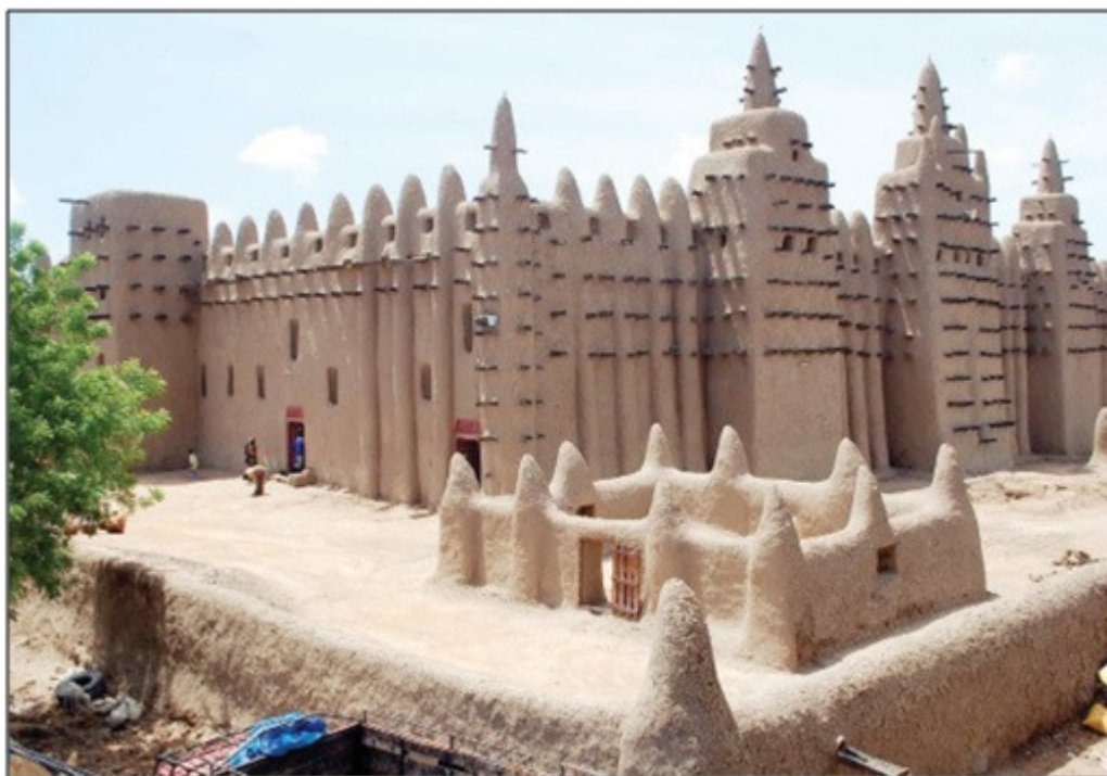
Plate 1: Djenne's Mosque, Mali-Largest Building Constructed of Mud Brick in the World Source: The Islamic Times: Way To Go Mali
