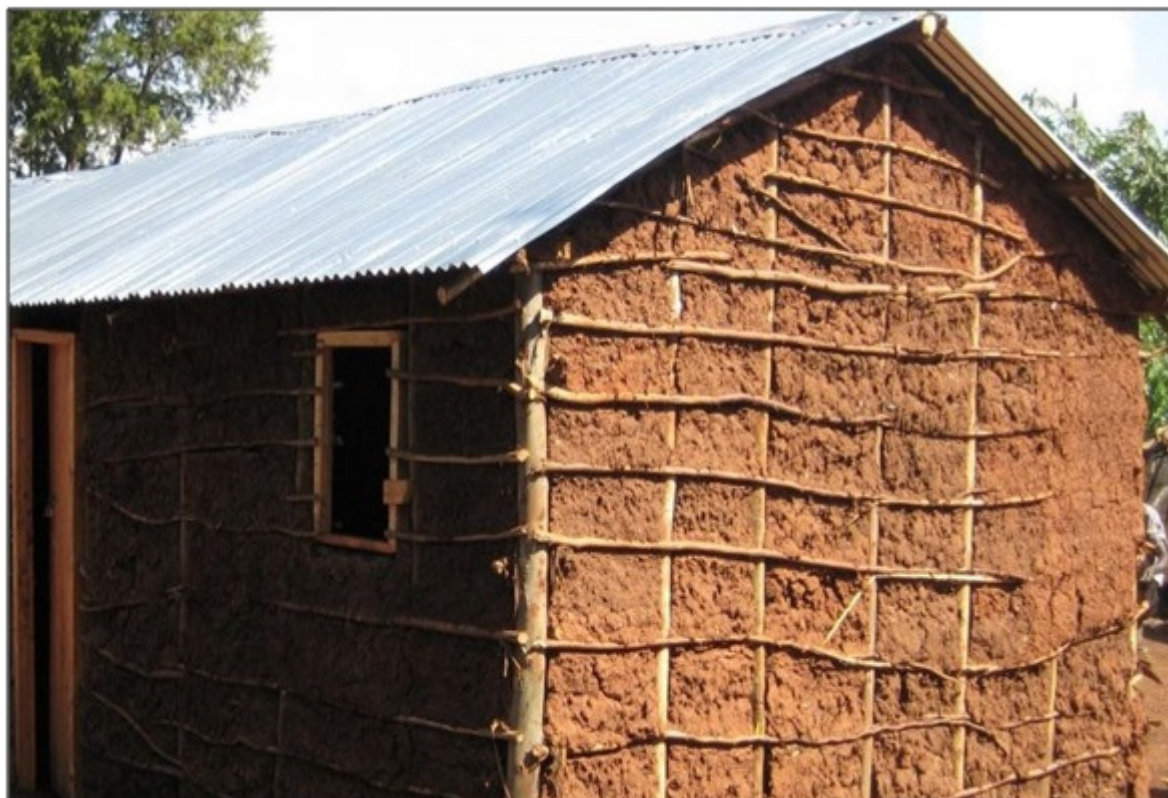
Plate 4: Wattle and Daub earth wall technique.
